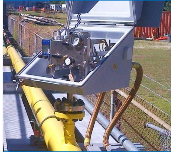
Figure 3 – GasPTi pipeline mounted installation
