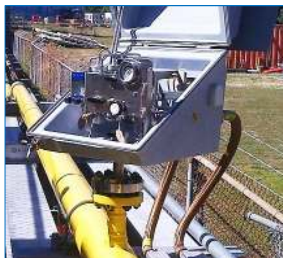
Figure 3 - PTi pipeline mounted installation
