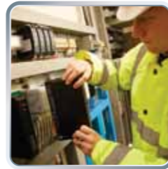
Insert replacement processor
